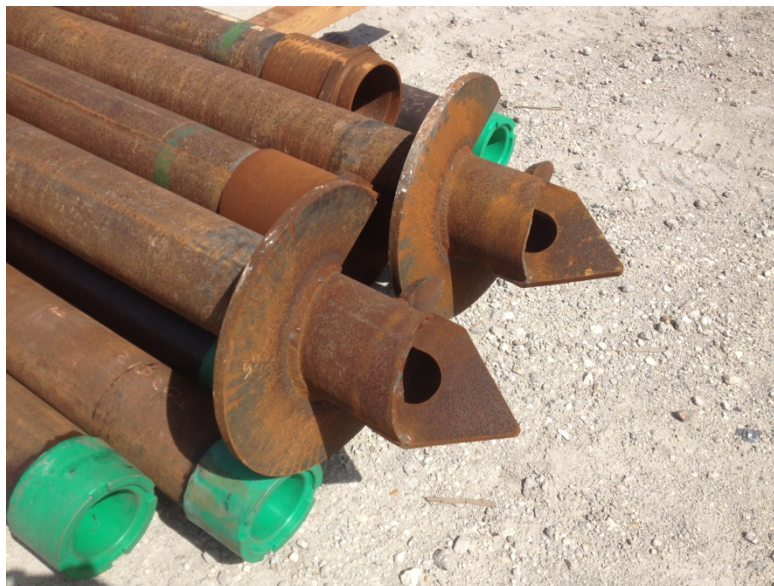
Photo 1 – Helical Pile Tip
