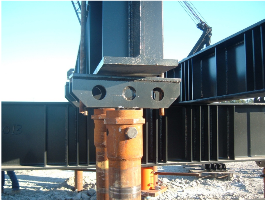
Photo 6 – Attachment of the Load Frame to the Anchor Piles
