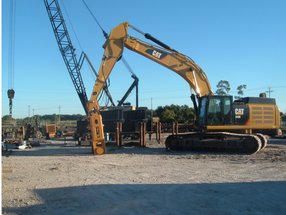
Photo 4 – Caterpillar 349E with the Rotery Pile Driving Head.
