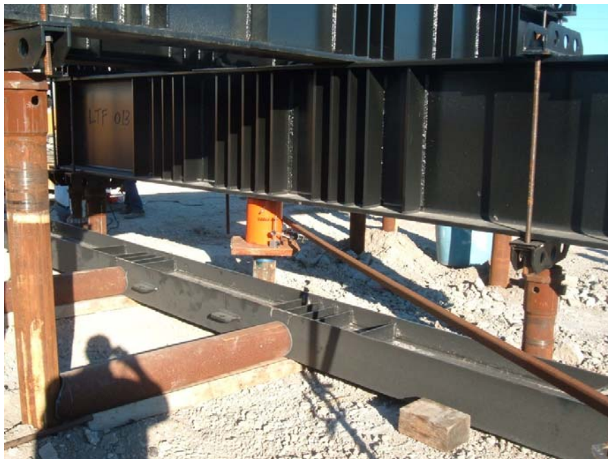
Photo 7 – Load Frame Setup for the Vertical Load Test
